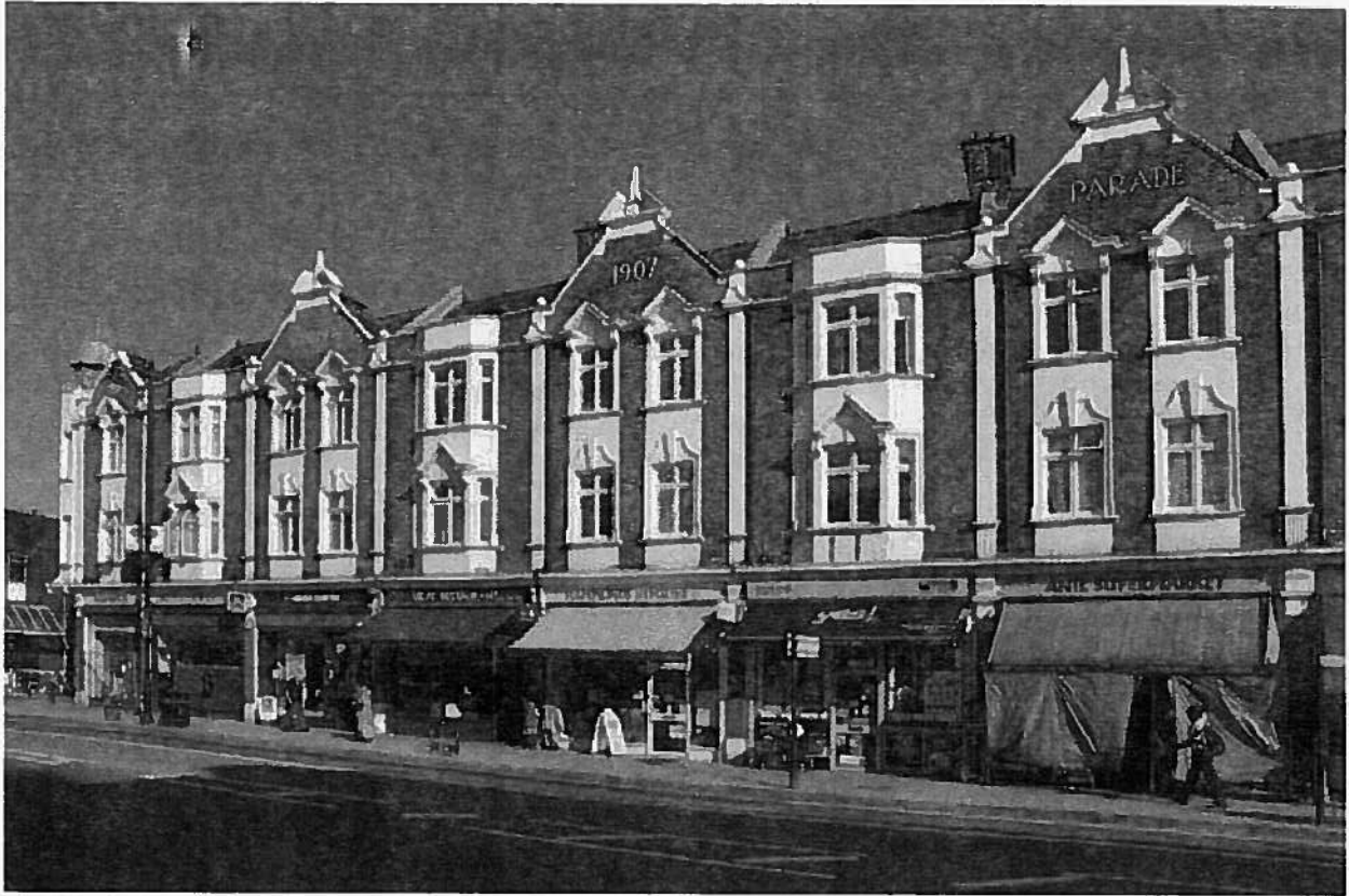
Completed LBH shopfront improvements scheme funded through EH.
