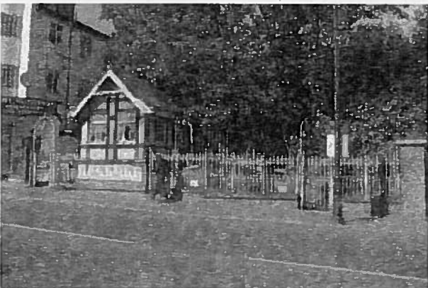
Bruce Grove Toilets - LBH have already done a feasibility study looking at how the toilets might be brought back into use. £25k has been secured from EH to restore the exterior. The borough is not asking for further funding from OLF for this project.
